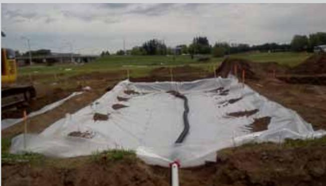
Excavated plot with plastic lining placed on the bottom and a drain to collect leachate.
